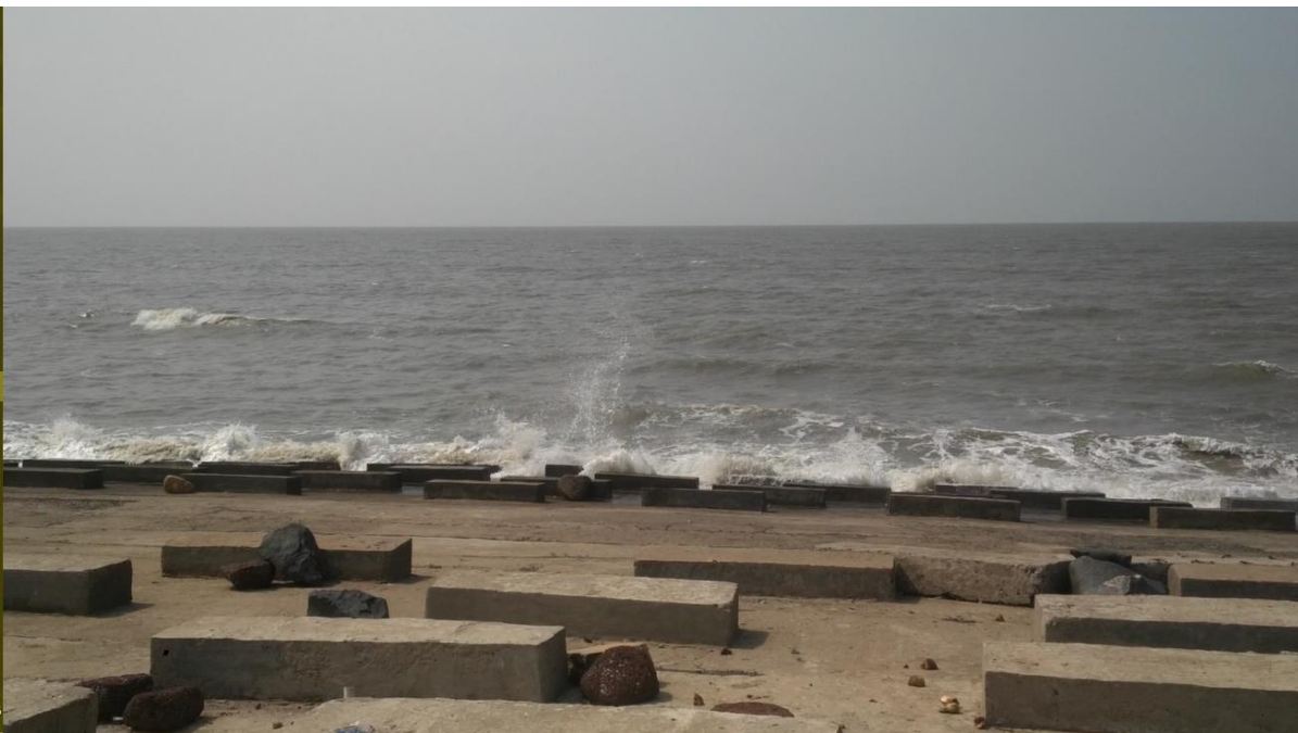
Photo 4.4.7 Waves breaking on Shankarpur Seawall at Low Tide
