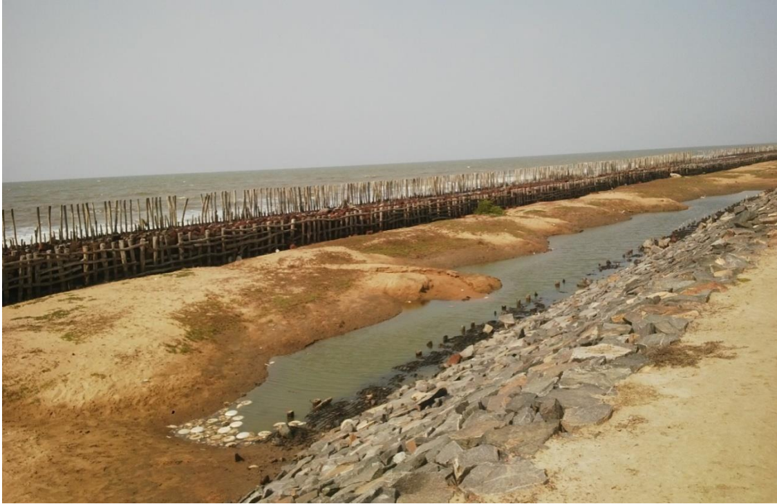
Photo 4.4.6 Shore Protection by pitching behind Timber pile seawall
