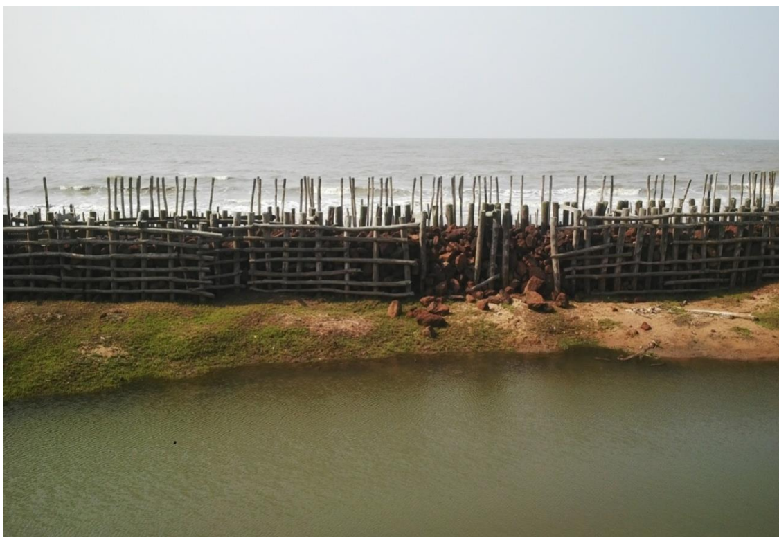
Photo 4.4.11 Seawall at Tajpur showing rubble fill between timber piles
