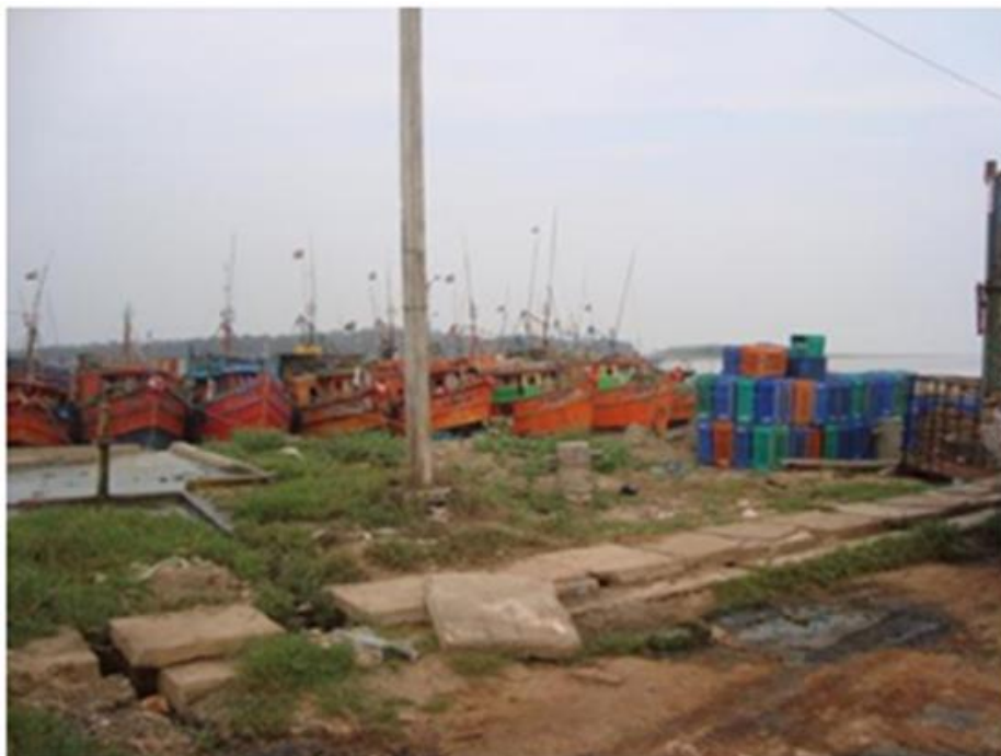
Photo 4.1.3 : Slipway construction at Petuaghat
