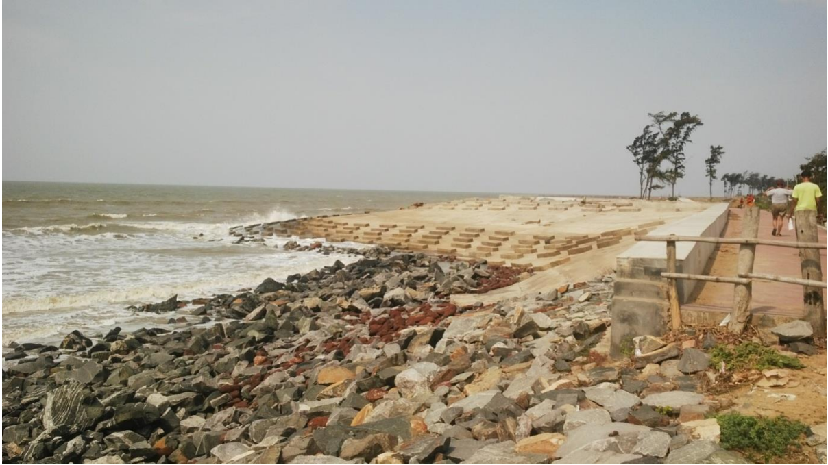
Photo 4.4.8: Shankarpur Seawall – Looking North from Tajpur
